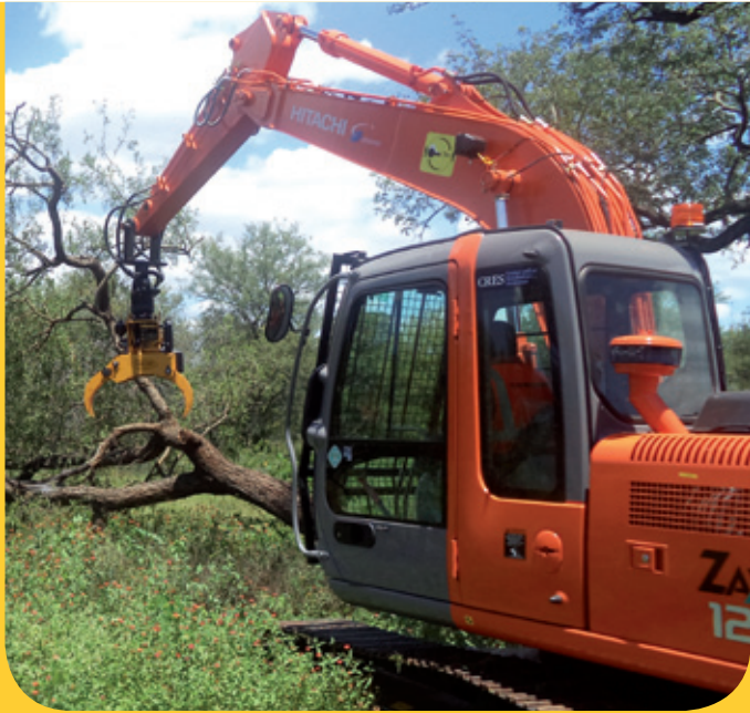
GMT035 on a Hitachi excavator
